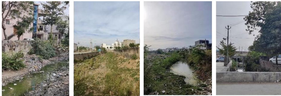
Fig 1: Current pictures of the canal
